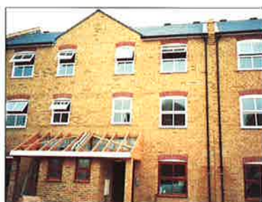
New build scheme at Halcroft Road E9 design & build contract
